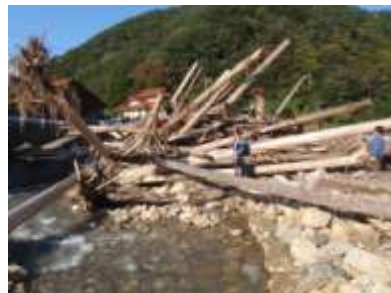
Figure 8. A back view of a woody debris accumulation at bridge without piers at Site 2 (taken from upstream of the river).
